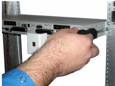
1. To begin installing the hinged pluggable back panel, the NetGuardian G5 should be rack mounted. **Suggestion:** Mount the unit in the flush, rack-mount position. This means the front of the NetGuardian is flush with the front of the rack post.
